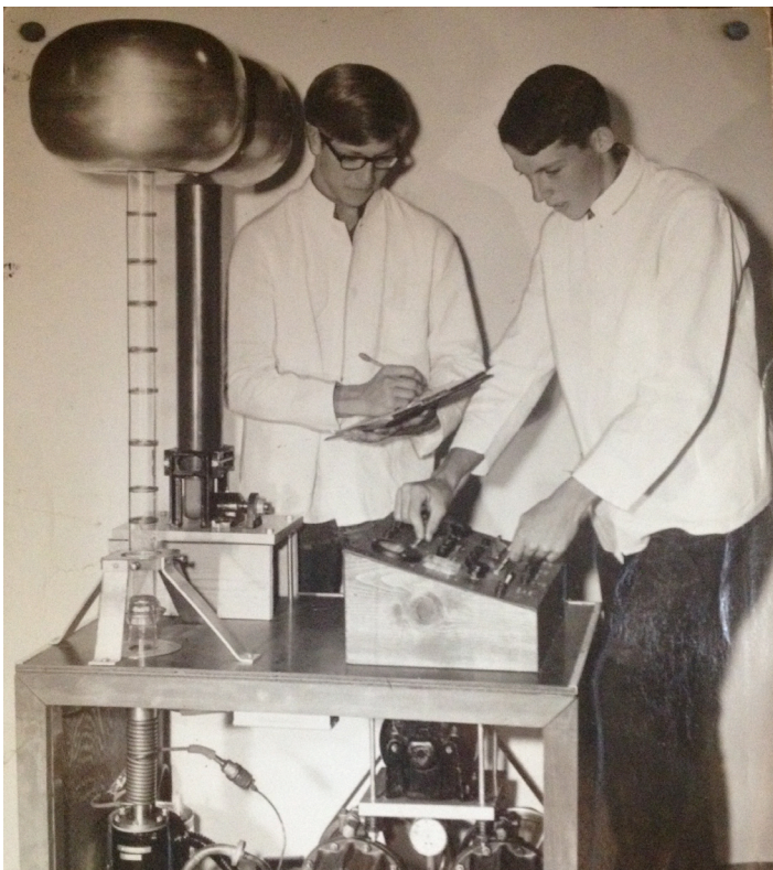
Patrick Edward with Jay Bernard building a Van de Graff generator electron particule accelarator
